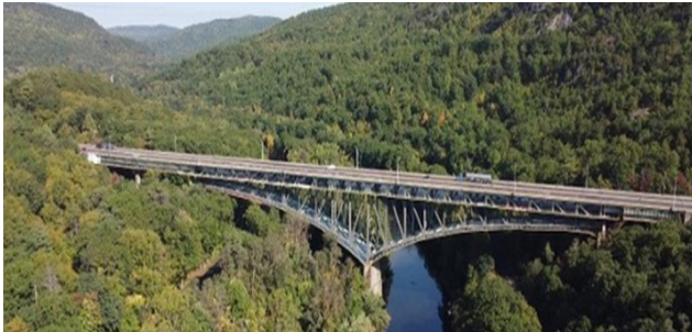
I-90 OVER WESTFIELD RIVER. 750-ft-long deck truss main span.
